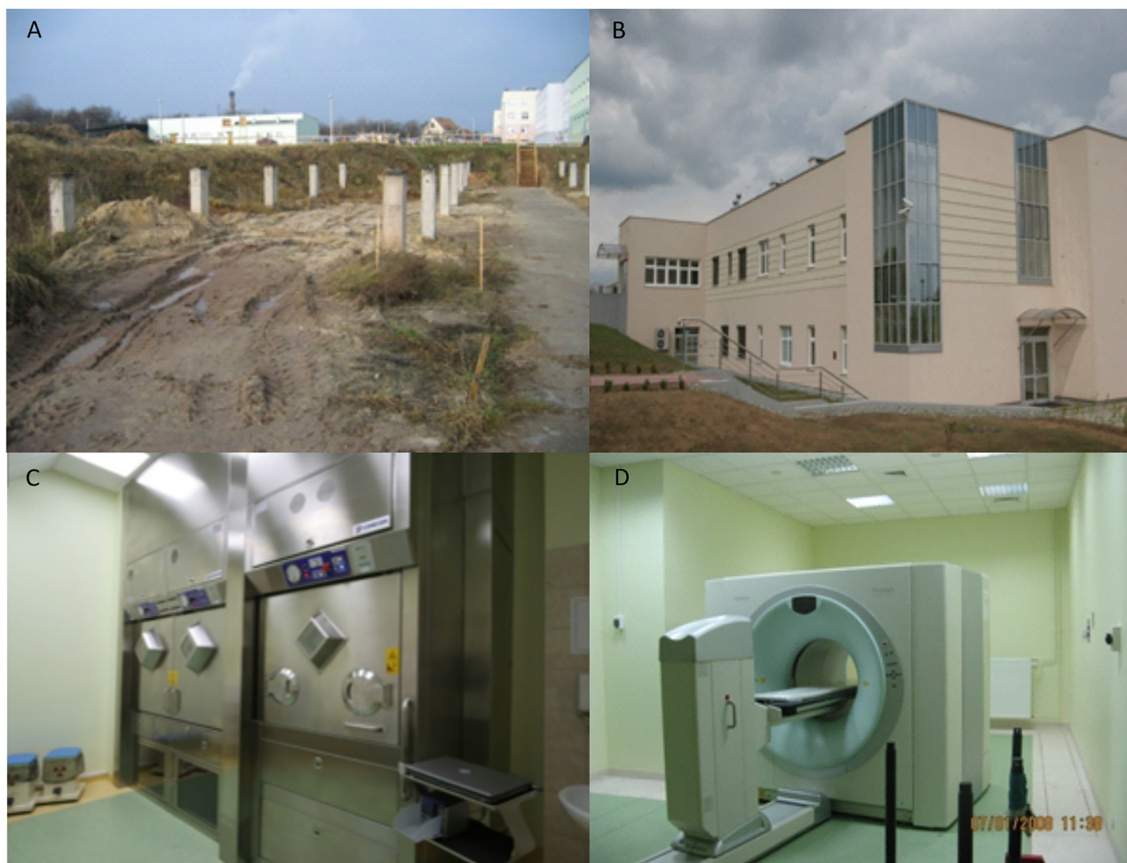
Figure 2: Beginning of the Department of Nuclear Medicine in the Holy Cross Cancer Centre: beginning of construction works, March 2007 (A); reception of the building, January 2008 (B); Dispenser, Comecer (C); PET/CT scanner (Biograph, Siemens) (D). Thanks to the Professor Janusz Braziewicz.
